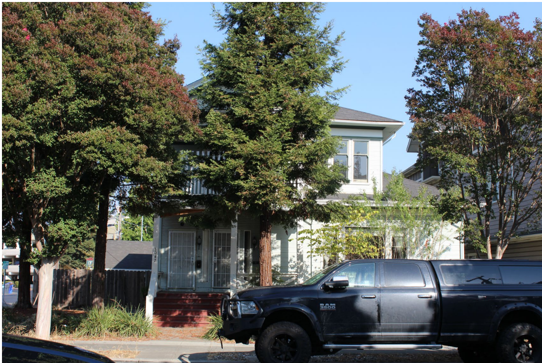
Photograph 2: West elevation, camera facing east
