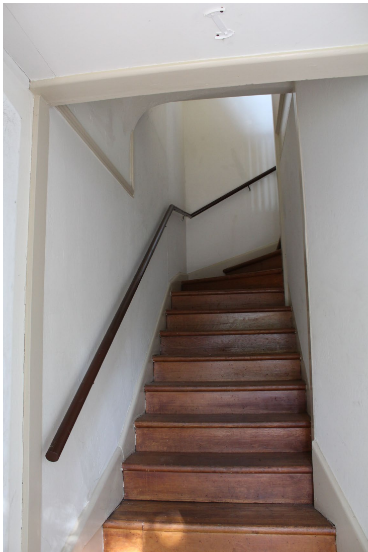
Photograph 15: Interior, entry stairs, camera facing east
