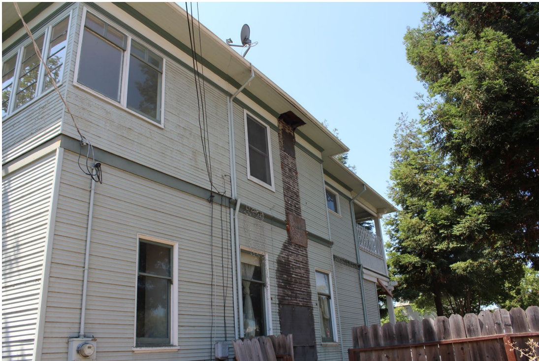
Photograph 6: North elevation, camera facing southwest
