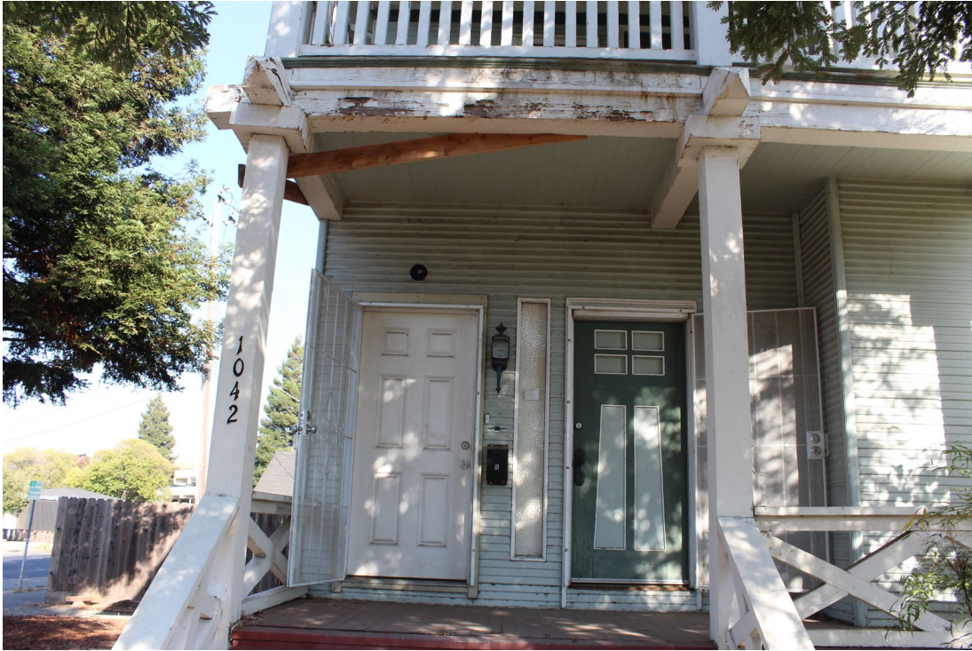
Photograph 3: Detail, main entrance and porch, west elevation, camera facing east
