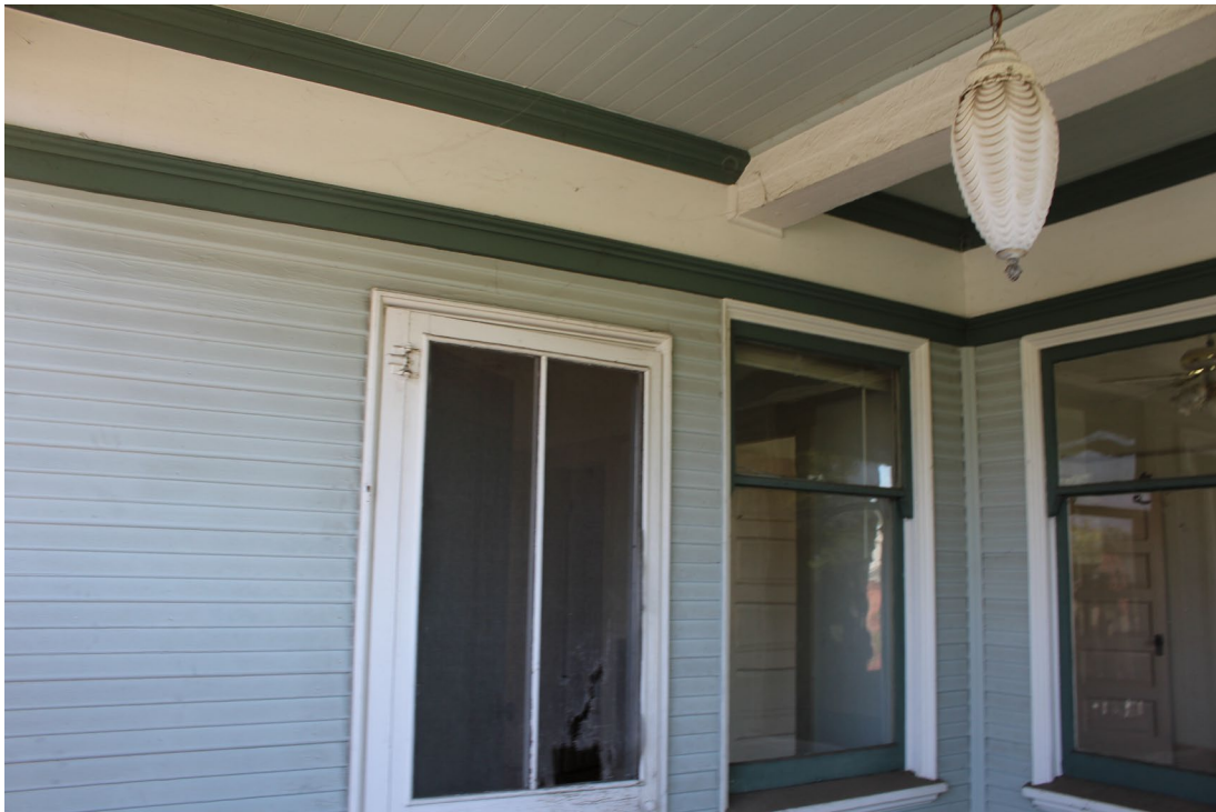
Photograph 4: Detail, second-floor balcony, west elevation, camera facing northeast
