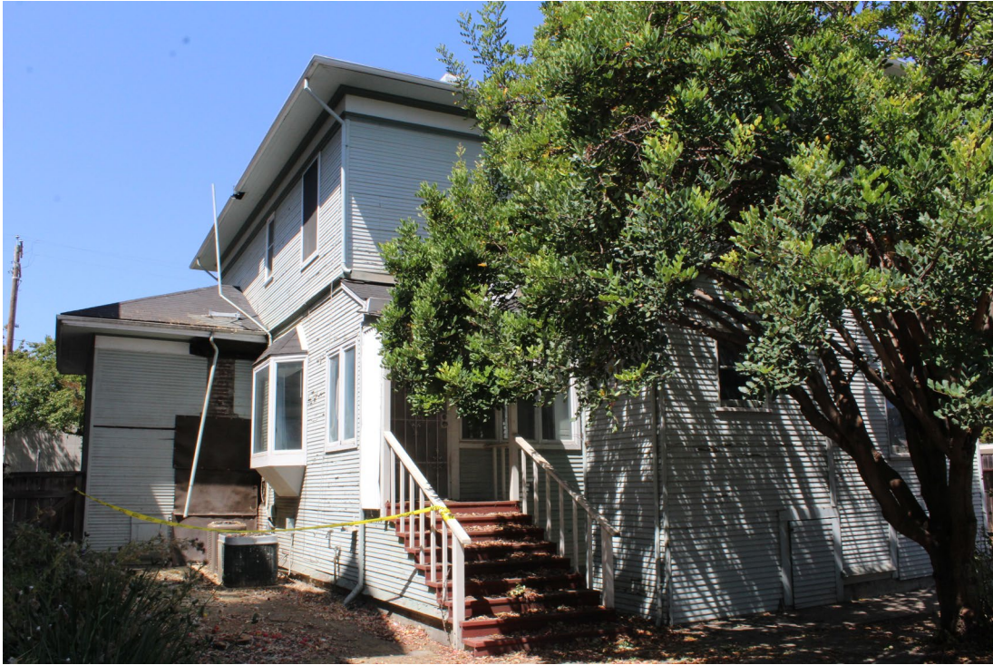
Photograph 7: East and north elevations, camera facing southwest
