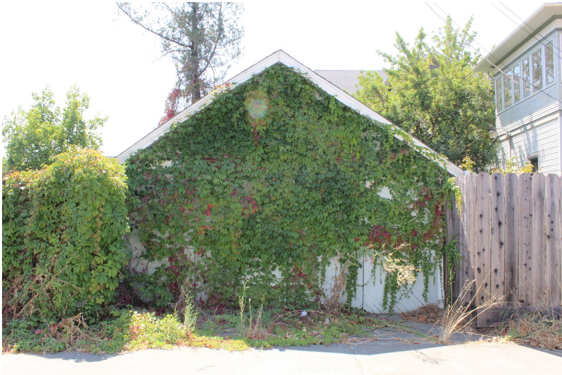
Photograph 8: Garage, north elevation, camera facing south
