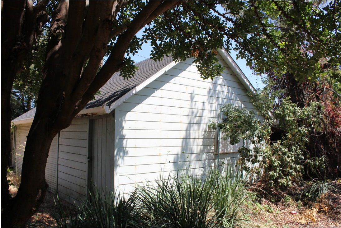
Photograph 9: Garage, west and south elevations, camera facing northeast
