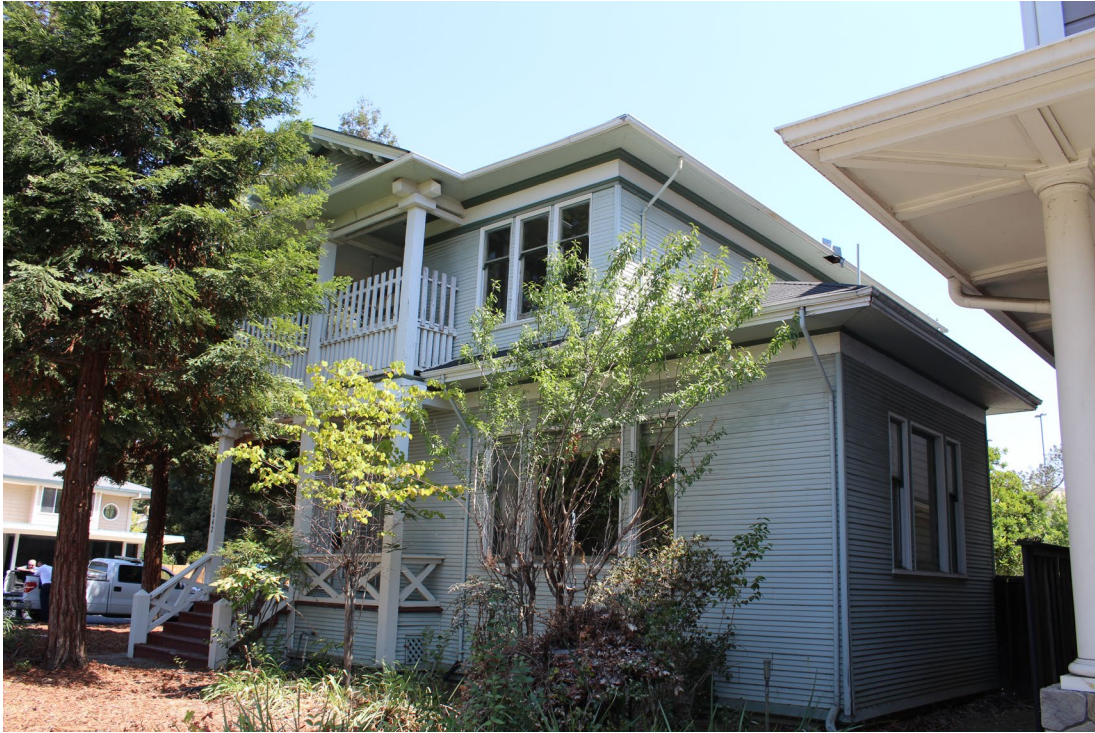
Photograph 1: West and south elevations, camera facing northeast
